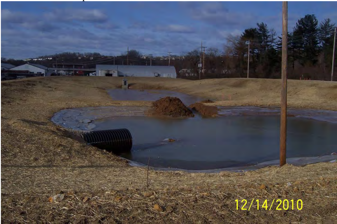
View looking west at finish grades for new stormwater detention pond.
