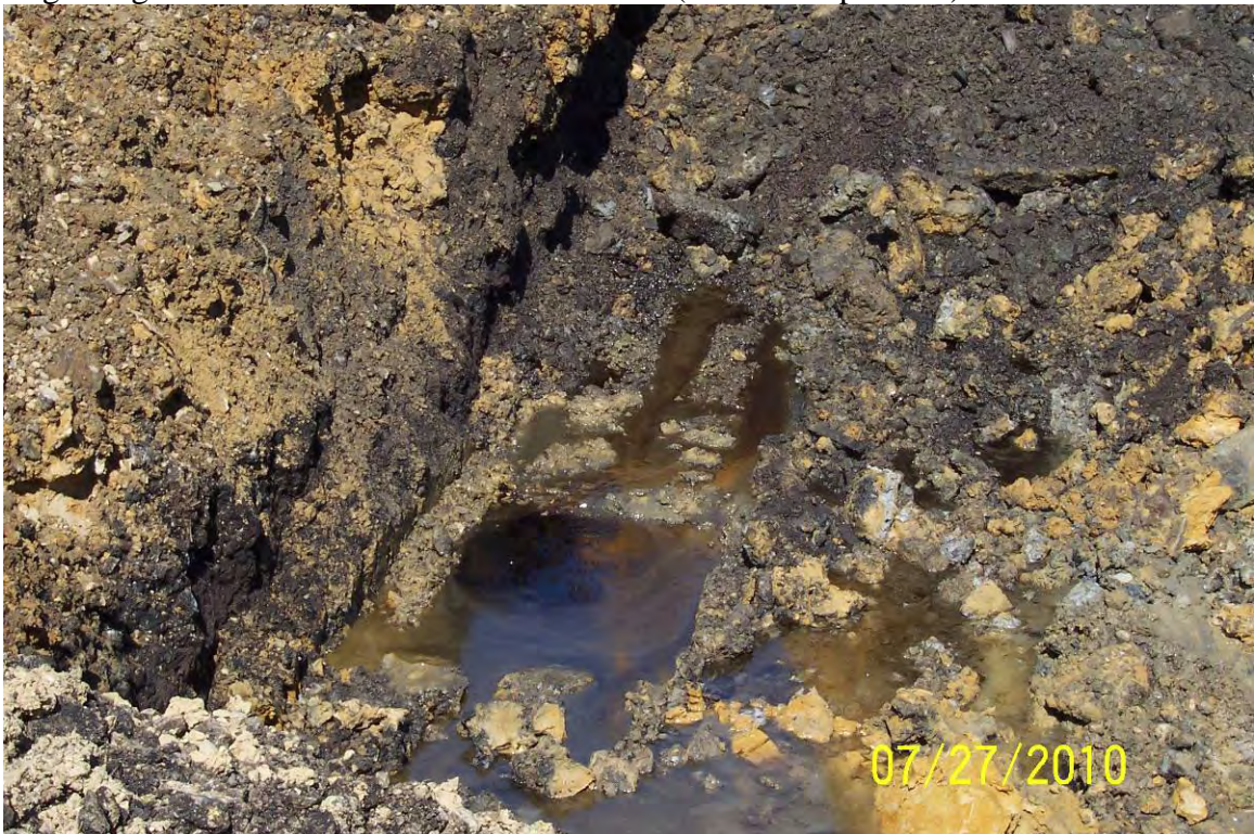
View looking south from railroad bed area just north of the former Metal Chip Bin area. Beginning of excavation – note oil on the water (see close-up below).
