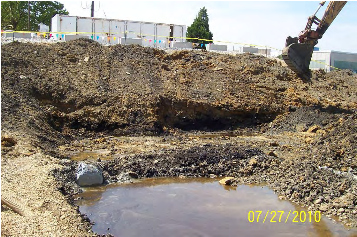
View looking south from railroad bed area just north of the former Metal Chip Bin area. Beginning of excavation – note oil on the water (see close-up below).
