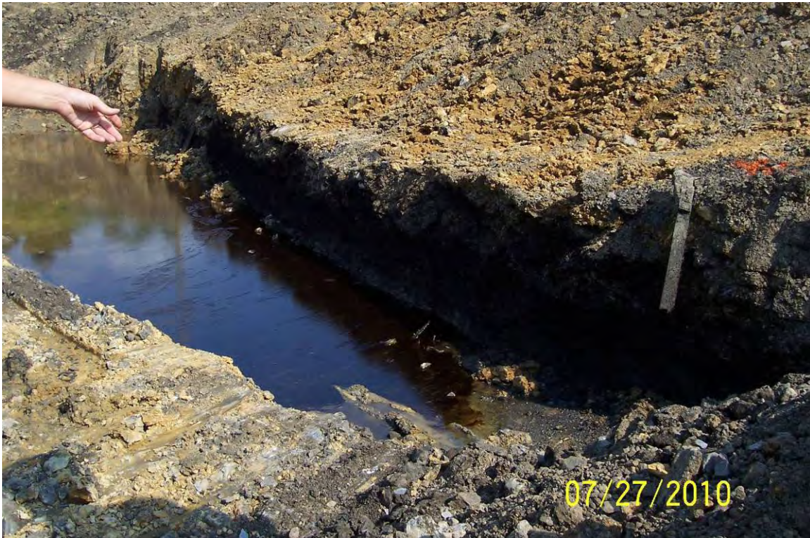
View of oily liquid and black soil found during initial removed from former Metal Chip Bin area.
