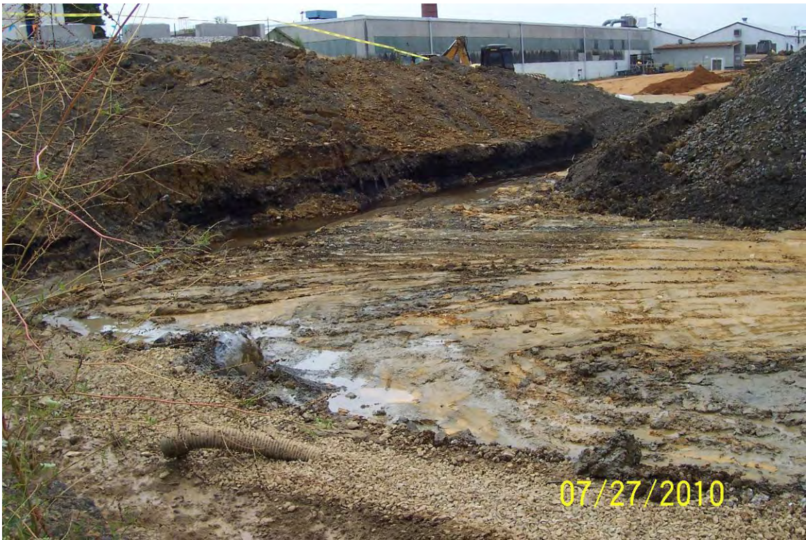
View looking southwest at area of soil removal in MCB area.
